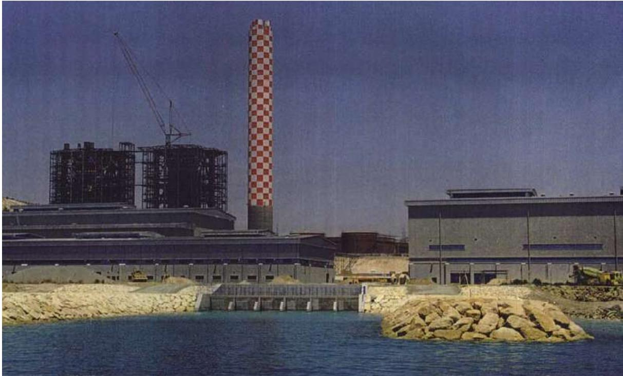
**Figure 4.1** The inshore cooling-water outfall of the Vasilikos power plant (Turnpenny et al. 2010).
